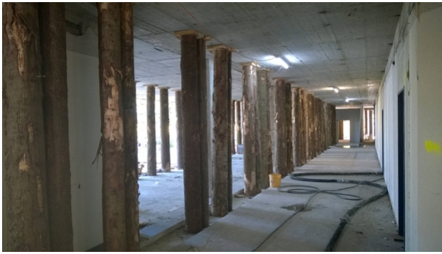
Temporary support with tree trunks
