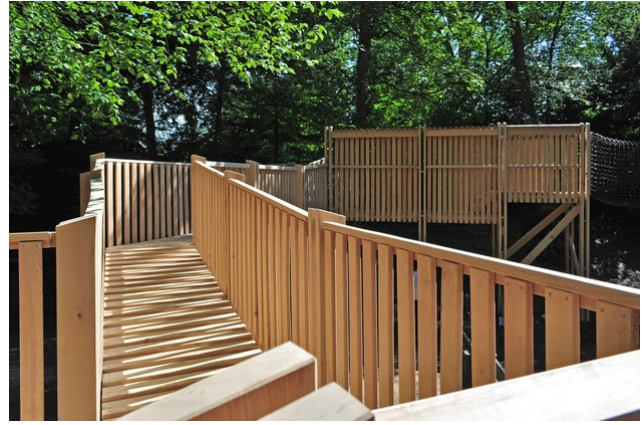
In keeping with the name, only beech wood was used for the Buchholz playground
