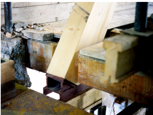
UNP beam, end support truss
