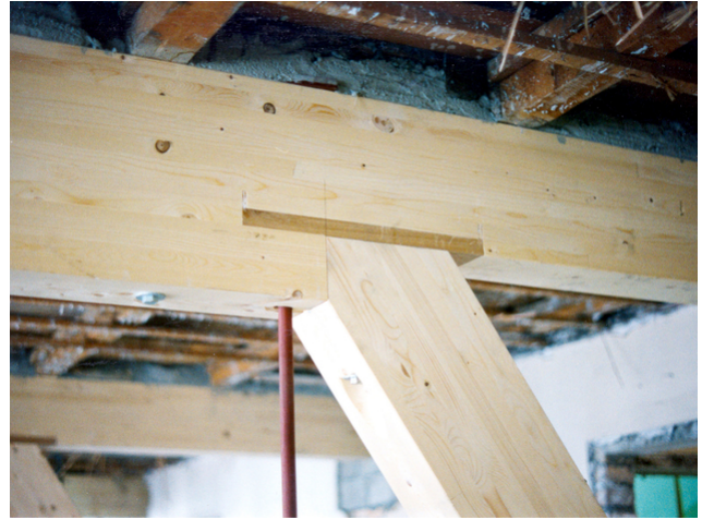
Transverse compression reinforcement with hardwood
