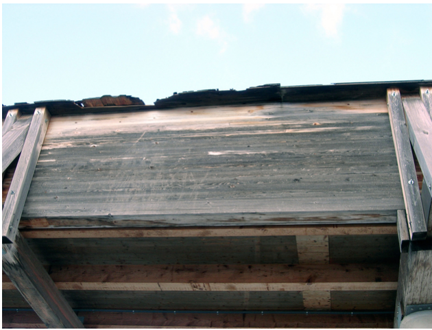
Pedestrian bridge before renovation 2
