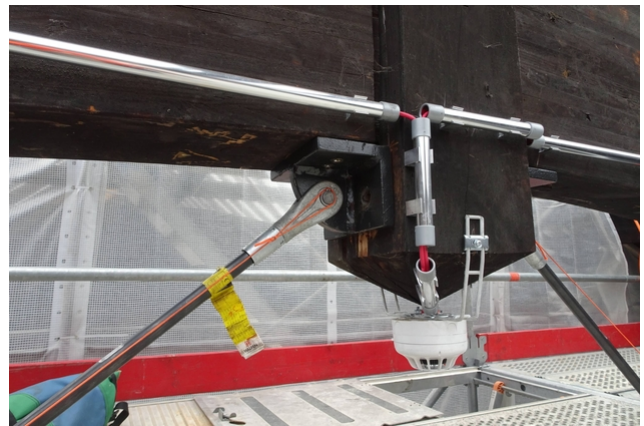
Fastening tie rods
