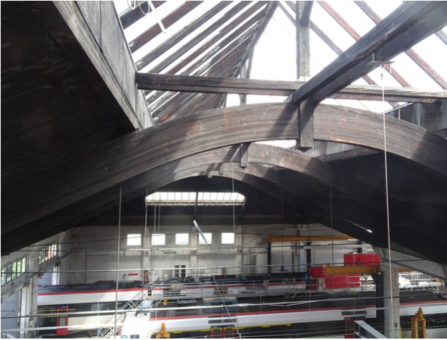
Arch truss with drawstrings
