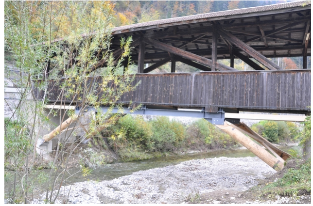
View of the bridge after renovation
