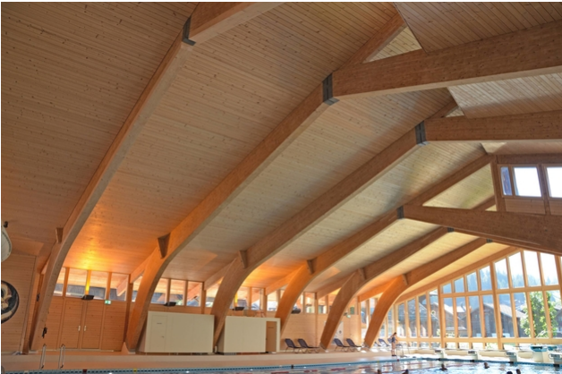
The beam on the far left is additionally reinforced with slats
