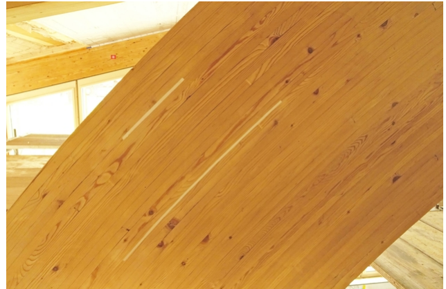
Detailed view of a rehabilitated adhesive joint
