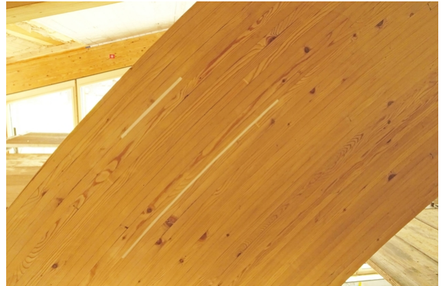
Detailed view of a rehabilitated adhesive joint
