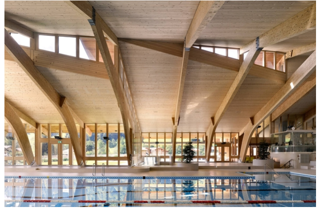
Between the trusses was renewed acoustic paneling
