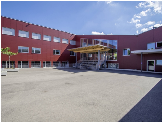
One unit: on the left you can see the gymnasium, next to it the connecting wing, on the right the renovated school building
