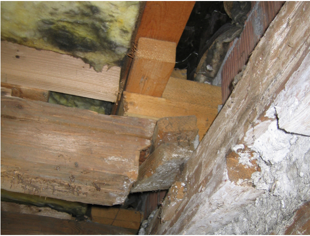
Beam support OG before renovation
