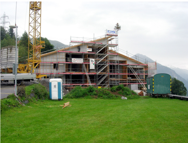
Shell of the building
