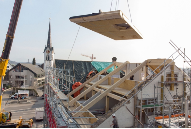
Attic conversion with the installation of prefabricated elements
