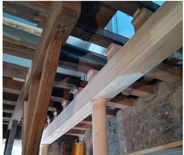
Renovation measures in the wine cellar
