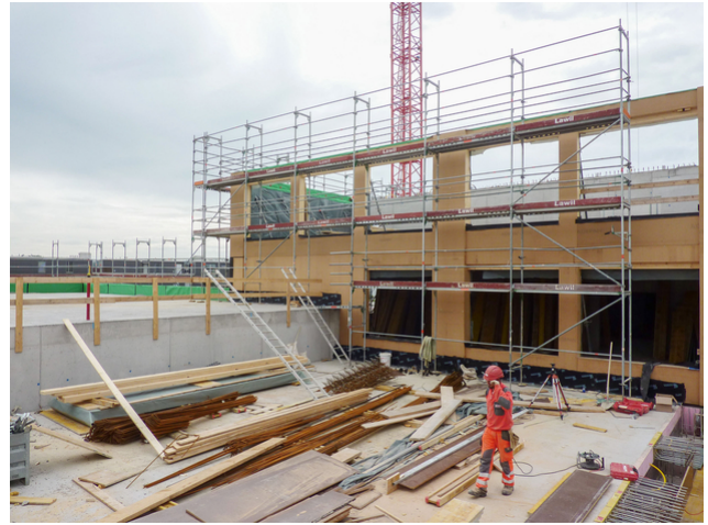
Wooden elements for the new school facility under construction
