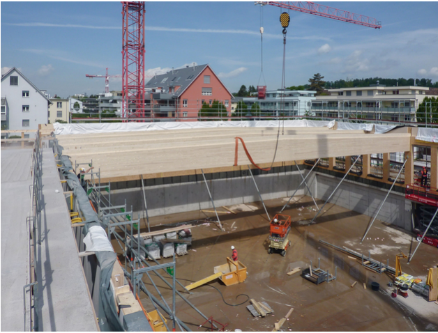
Installation of roof racks for the new sports hall
