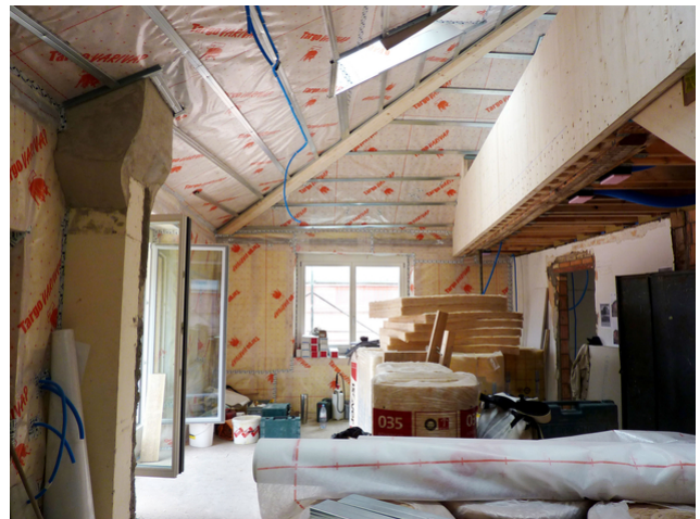
Living space during renovation
