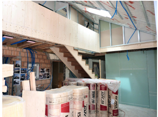
Kitchen during renovation
