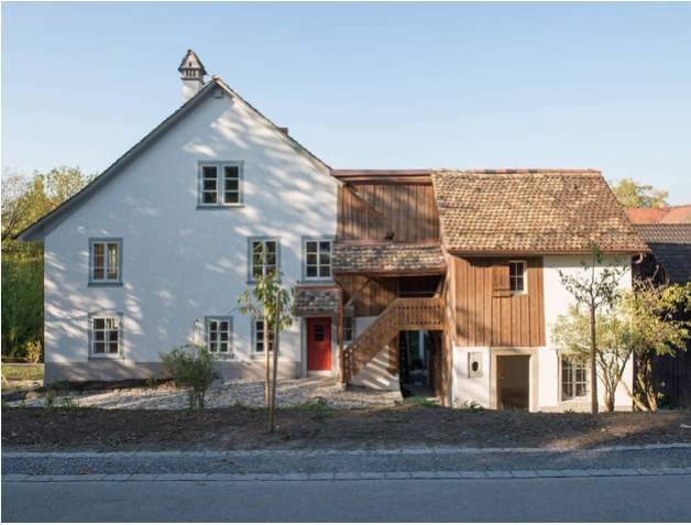
View from the street side
