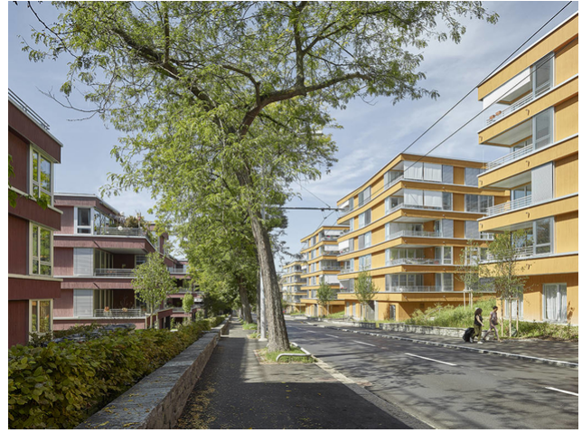
Road side 1st and 2nd stage
