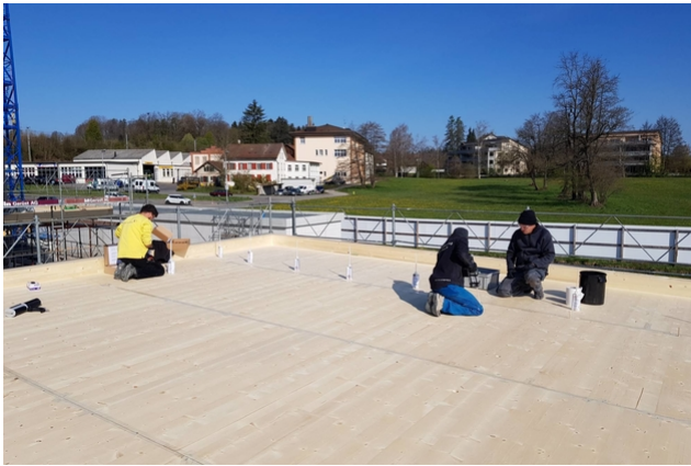
TS3 during TS3 grouting of the canopy
