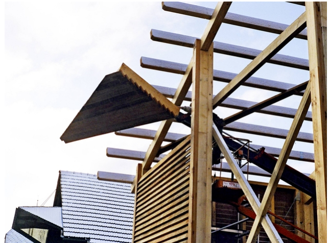
Assembly of the wall elements
