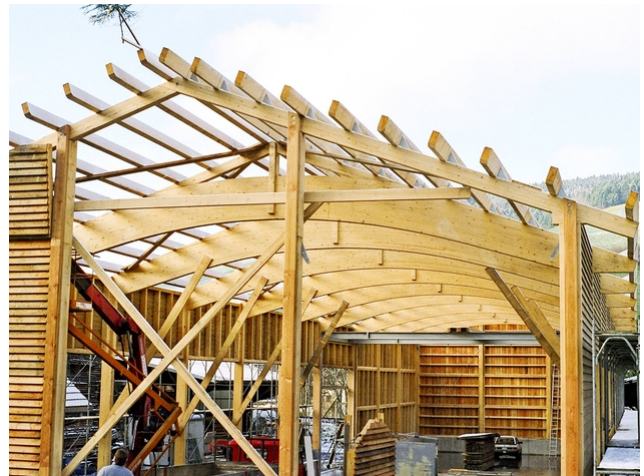
Assembly of the wall elements
