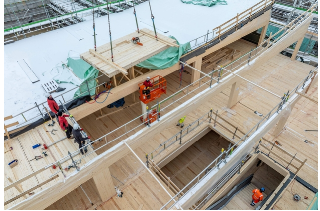
The extensive wooden room program is being erected
