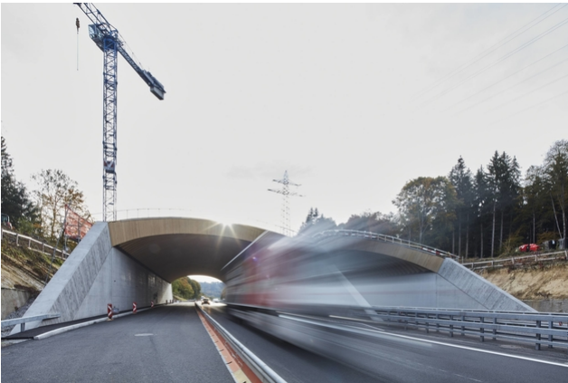
Assembly work during the day
