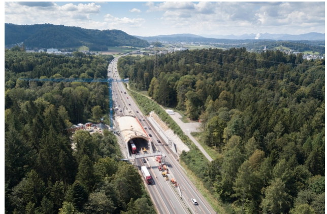
Aerial view during assembly
