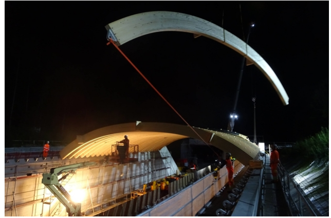
Assembly work at night
