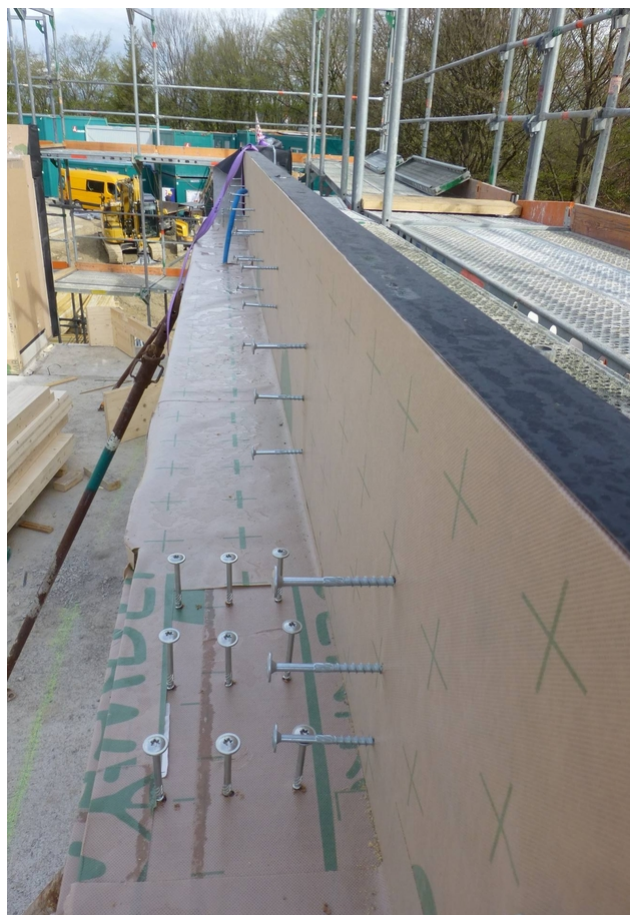
End formwork with column connection
